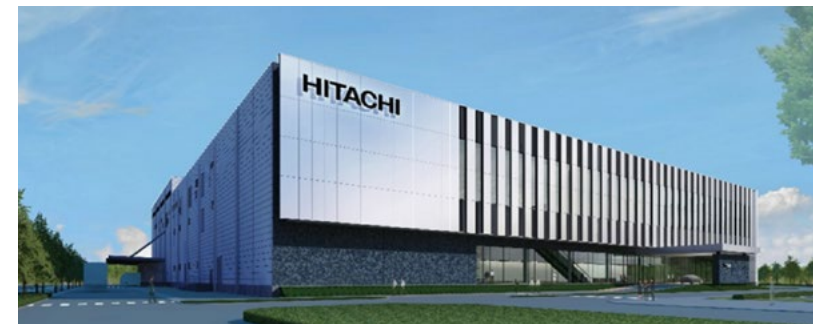
New manufacturing building at Hitachi High-Tech's Kasado Area (image of completion)
