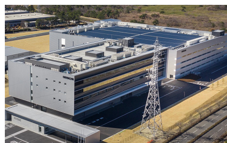
Naka Marine Site rooftop solar panels
